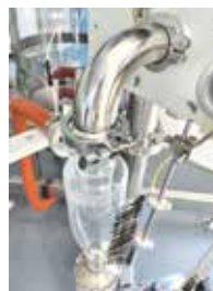
The cyclone separation unit is equipped with a safety cover to prevent burns and an anti-static brush.
